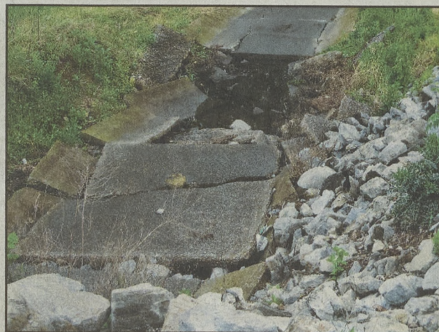
PRESS PHOTO BY BERNIE O'HARE A concrete liner for stormwater drainage to Monocacy Creek needs a little work.
