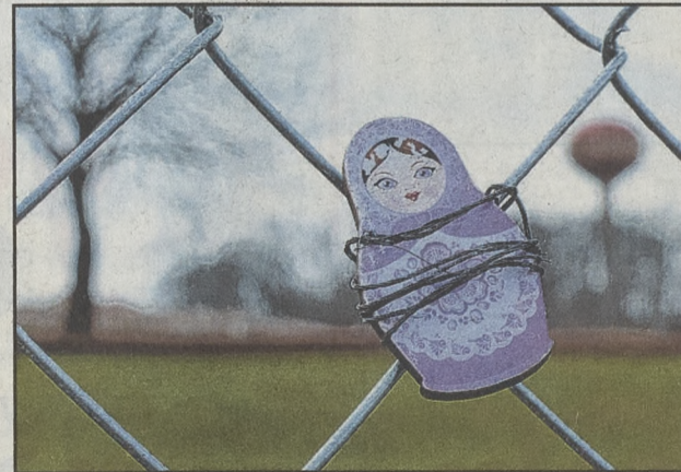
A memento resembling a Russian nesting doll is attached to the temporary chain link fence around the demolition site.
