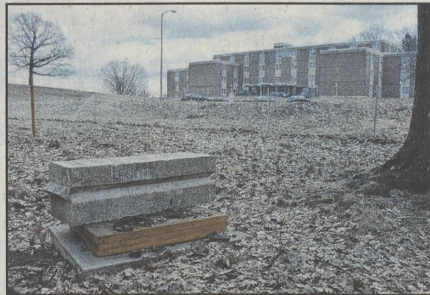
Heavy weights are placed atop a tunnel shaft to prevent access. In the background is the hospital's administration and admissions building, erected in 1969.
