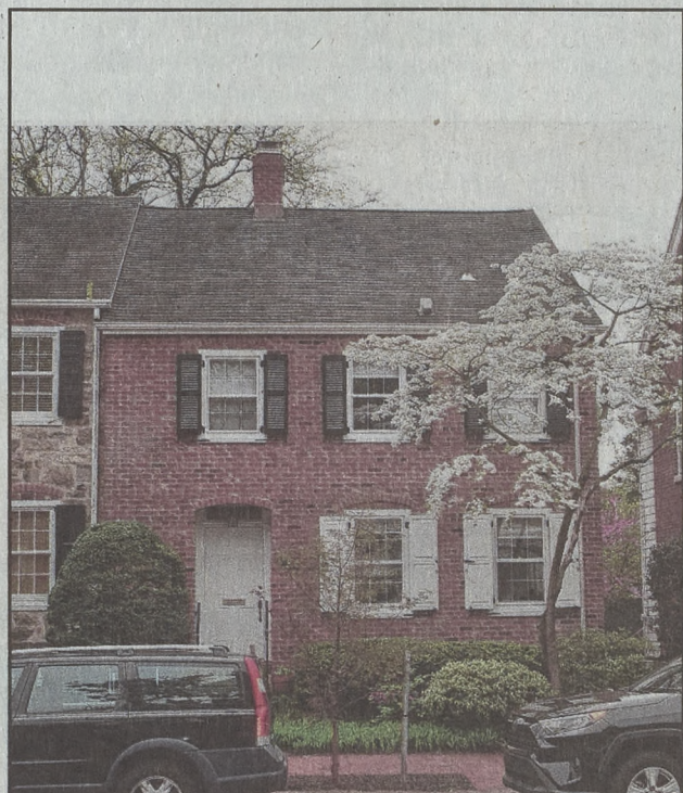
Replacement roofing and windows were approved for 52 E. Wall St., owned by Donald and Elke Rockwell.
