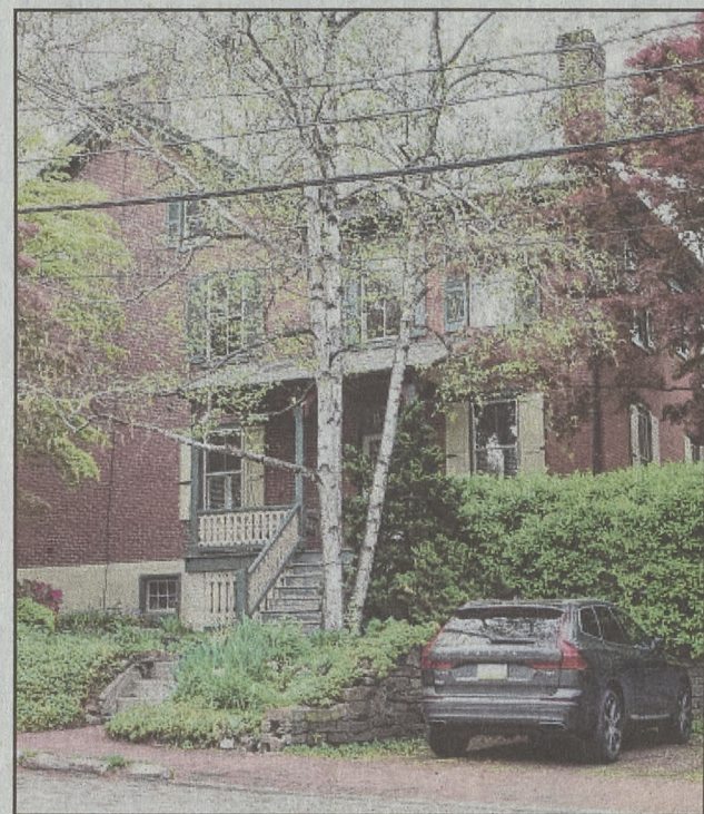
The Carnahans' corner property at 444 N. New St. is shown facing Wall Street. The couple proposes replacing concrete stairs with flagstone and resurfacing their parking pad.
