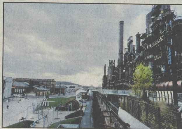
The ArtsQuest SteelStacks campus, celebrating its fifth anniversary this summer, includes the TD Community Stage at Air Products Town Square, Levitt Pavilion SteelStacks, Visitor Center and Hoover-Mason Trestle.
