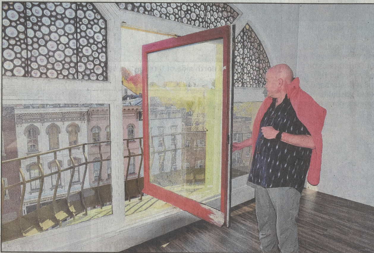
Owner Jay Brew demonstrates a swivel window at one of the upper floor balconies. The 'bullet' glass in this window is original to the building. More photos on A2. Story continues on A3.
