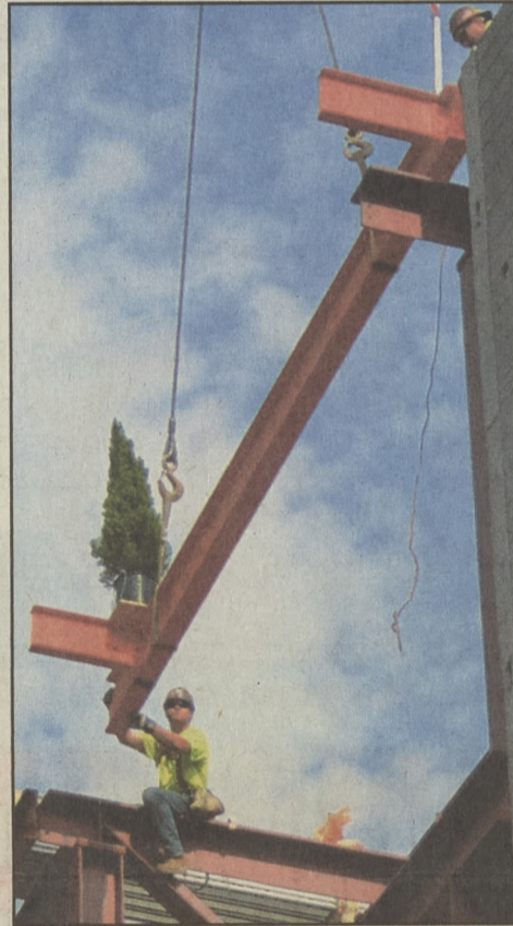
In mere minutes the great I-beam is hoisted over the heads of spectators and put in its place by steelworkers. The small tree tied to the beam's left corner signifies a project completed without accident to the crew.
