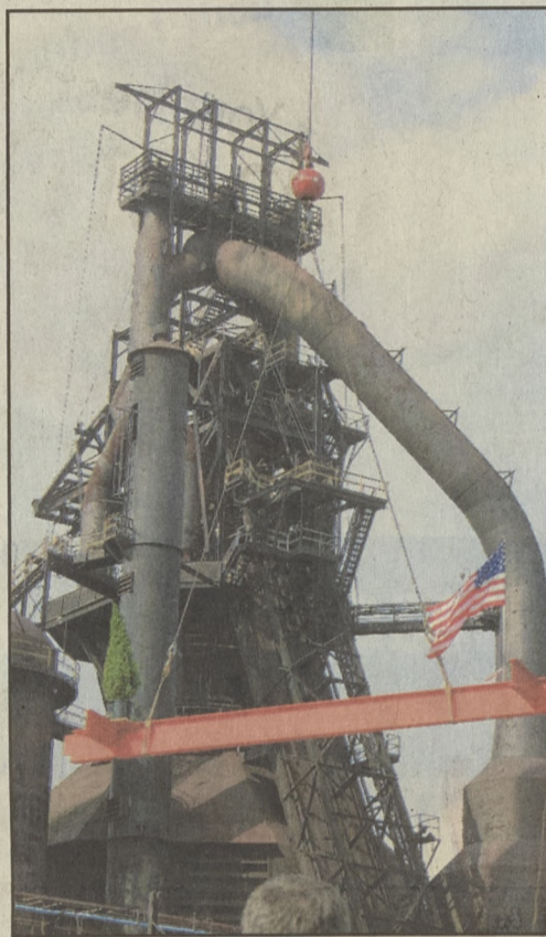
In mere minutes the great I-beam is hoisted over the heads of spectators and put in its place by steelworkers. The small tree tied to the beam's left corner signifies a project completed without accident to the crew.
