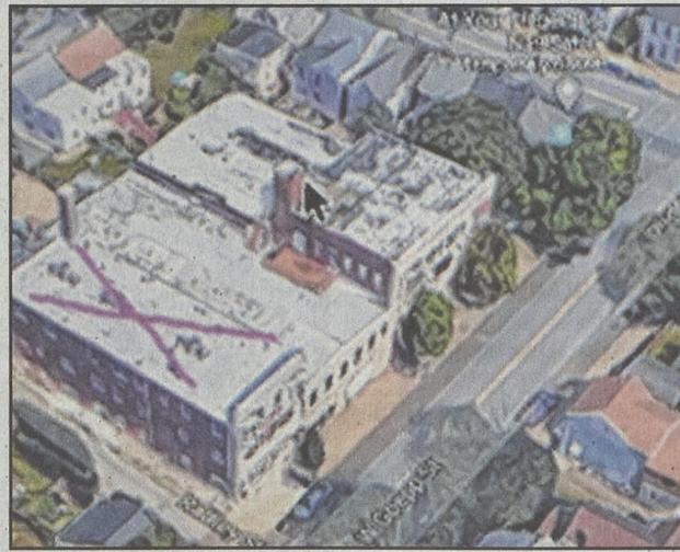
PRESS PHOTOS BY LANI GOINS 10-16 Goepp St. The pink "X" marks a building owned by another party. The other two portions of the building are the site for the planned apartments and office.
