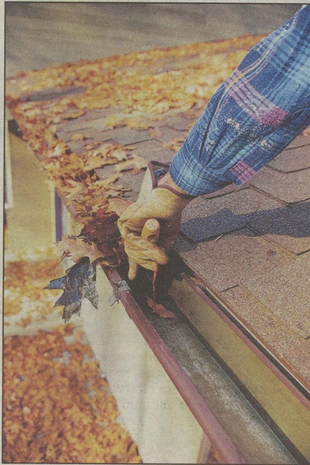
Cleaning gutters in the fall can prevent roof damage resulting from winter rains and snowfall.
