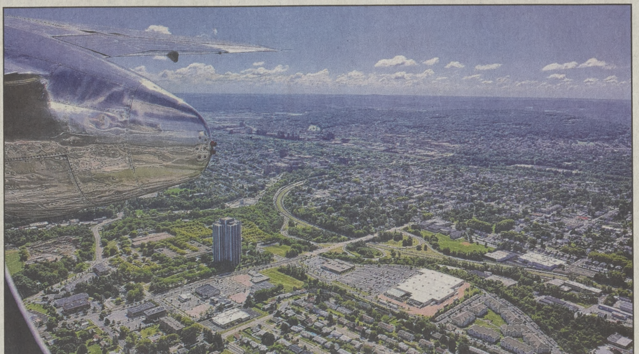
Former Bethlehem Steel world headquarters, Martin Tower , is below the B-25's starboard wing and South Mountain rises above Bethlehem in the distance.
