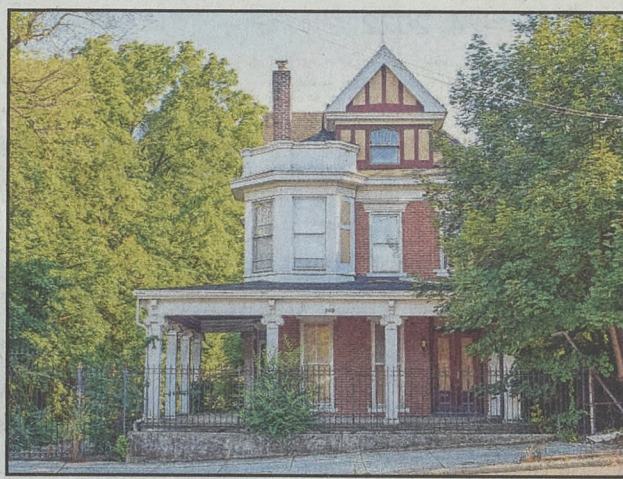
The demolition of this circa 1905 brick house at 143 W. Broad St. had been opposed by HARB, but approved by City Council in 2018.
