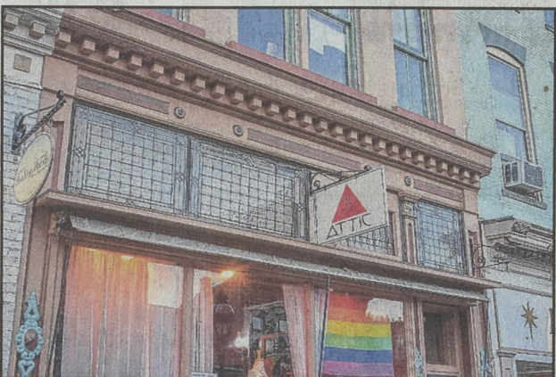
The approved non-illuminated blade sign for 516 Main St. will hang on the empty bracket at right.
