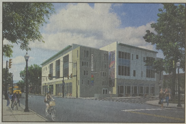
The new 87,000-square-foot Lehigh Valley Charter HS for the Arts will be constructed at East Third and Polk streets at a cost of $27 million.
