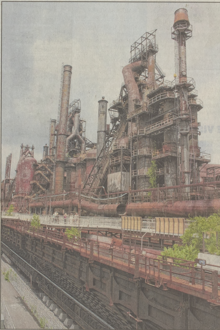
Even as visitors along the trestle tower over their surroundings, the immensity of Bethlehem Steel Corps' old furnaces looms behind them.
