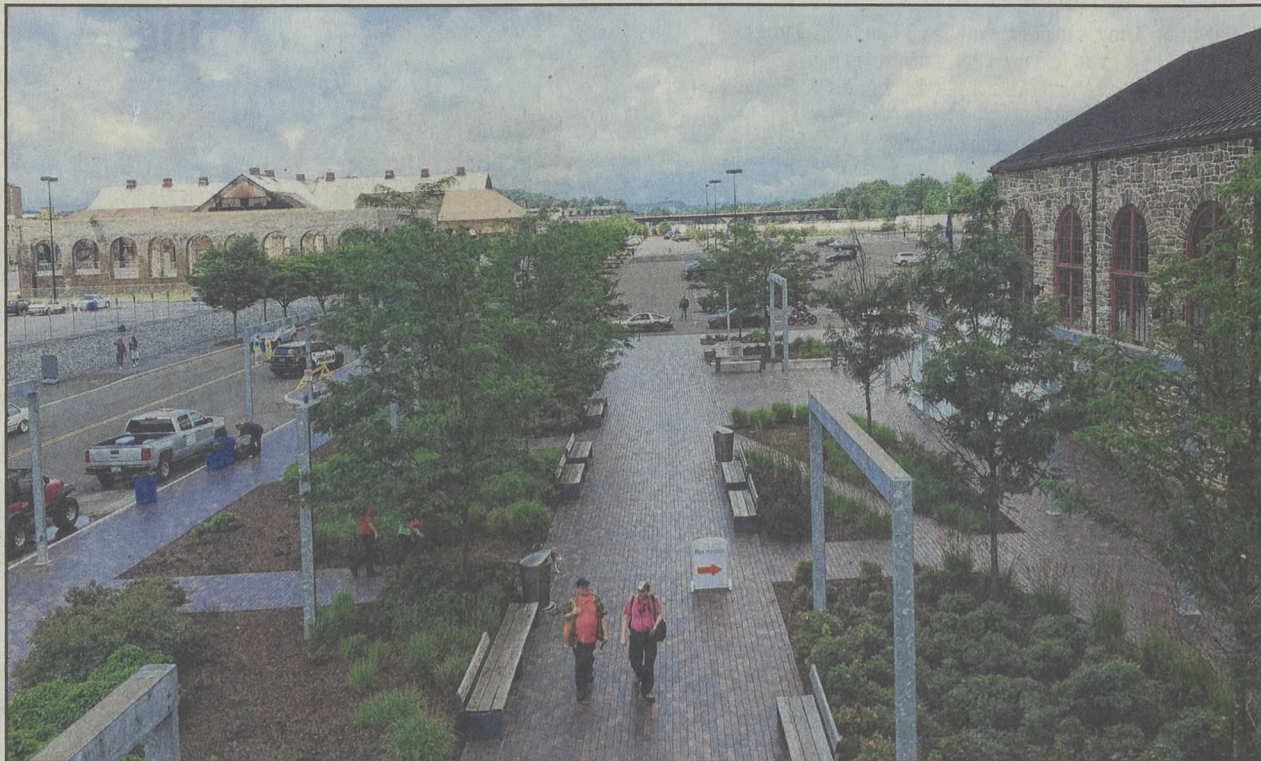
Looking west from the trestle - the Hill-to-Hill Bridge is in the background.
