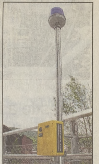
Emergency call boxes with flashing lights are placed intermittently to make certain help isn't far off.
