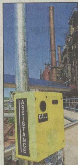
Emergency calling boxes ensure safety along the walkway of the Hoover Mason trestle at the former Bethlehem Steel blast furnaces.
