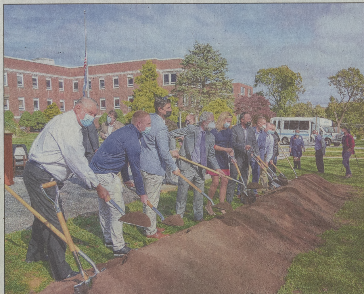
Lehigh County Director of General Services Richard Molchany and other invited guests shovel a spade of dirt, symbolizing the beginning of the construction phase of the new wing for Cedarbrook Senior Care and Rehab.
