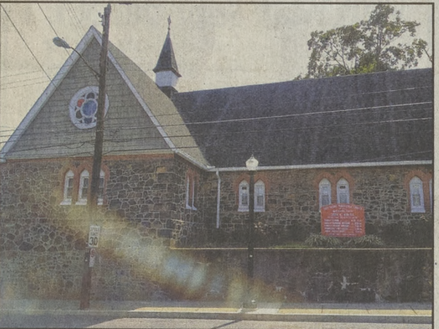
Built in 1884 for the Episcopal Mission of St. Joseph's Chapel, it now serves the Holy Bethel Pentecostal Church.
