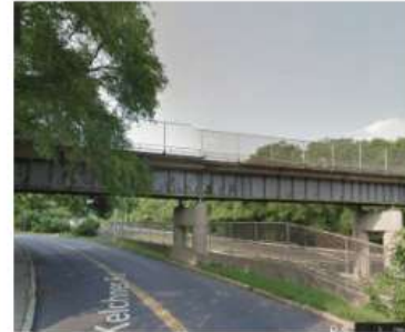
Existing RT 378 overpass
