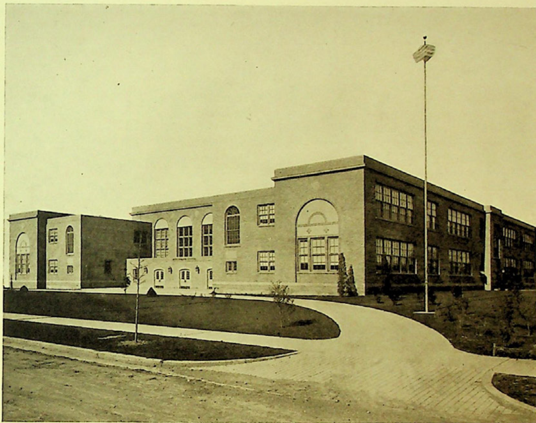
THE NITSCHMANN BUILDING
