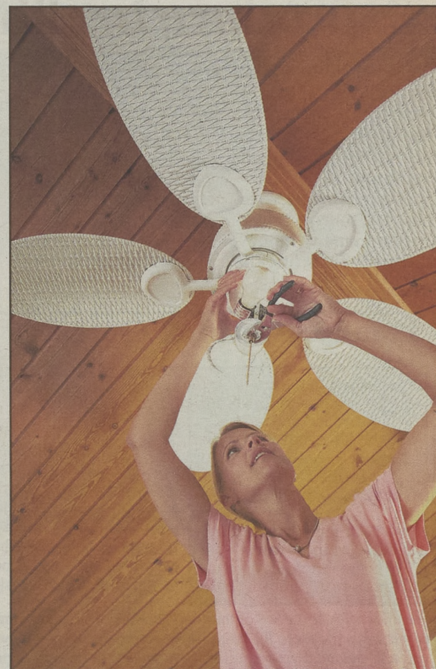
Ceiling fans can help cool a home more efficiently when fan blades spin in the right direction for the season.
