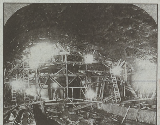
The Davies & Thomas Foundry provided the lining for this tunnel. In 1900, the excavated tunnel for the Interborough Rapid Transit is supported with scaffolding. IRT began operation Oct. 27, 1904, running from City Hall up to 145th Street.
