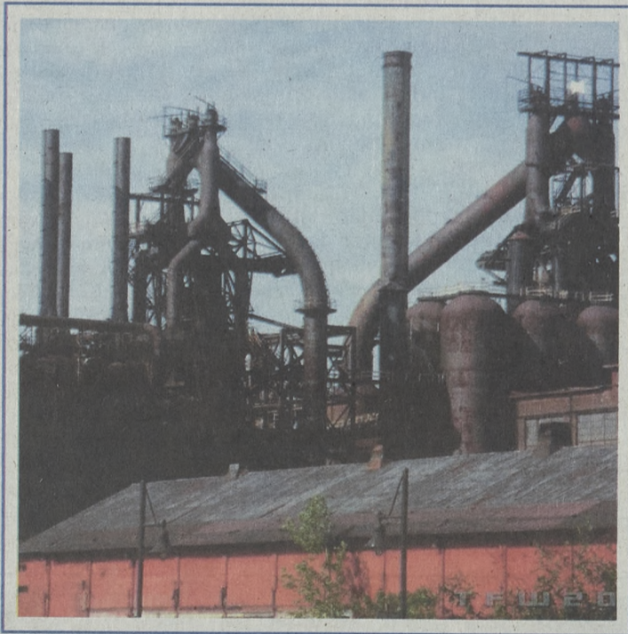
Steel Stacks - Bethlehem
