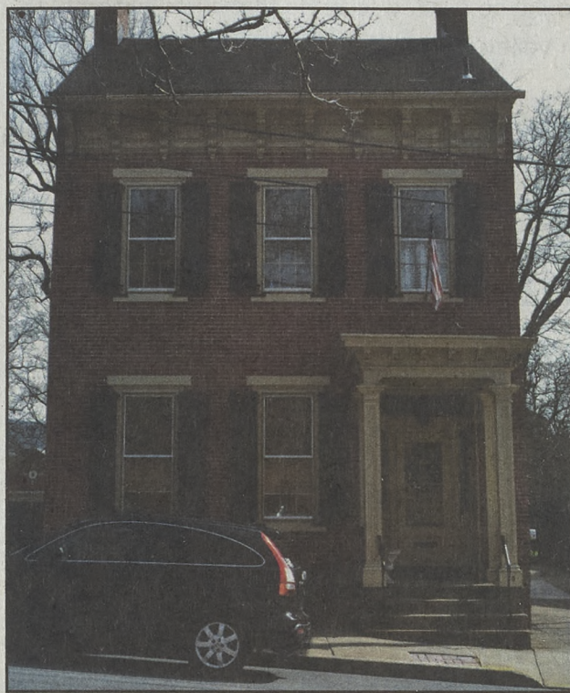
Roofing replacement with GAF Slateline shingles in antique grey was approved by phone with the contractor for 55 W. Market St.
