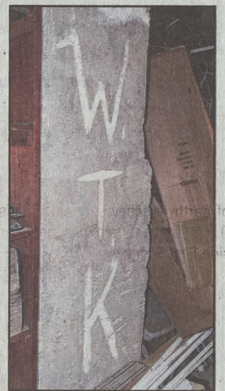
Renovations exposed drugstore owner William Kostas' initials on a basement column.
