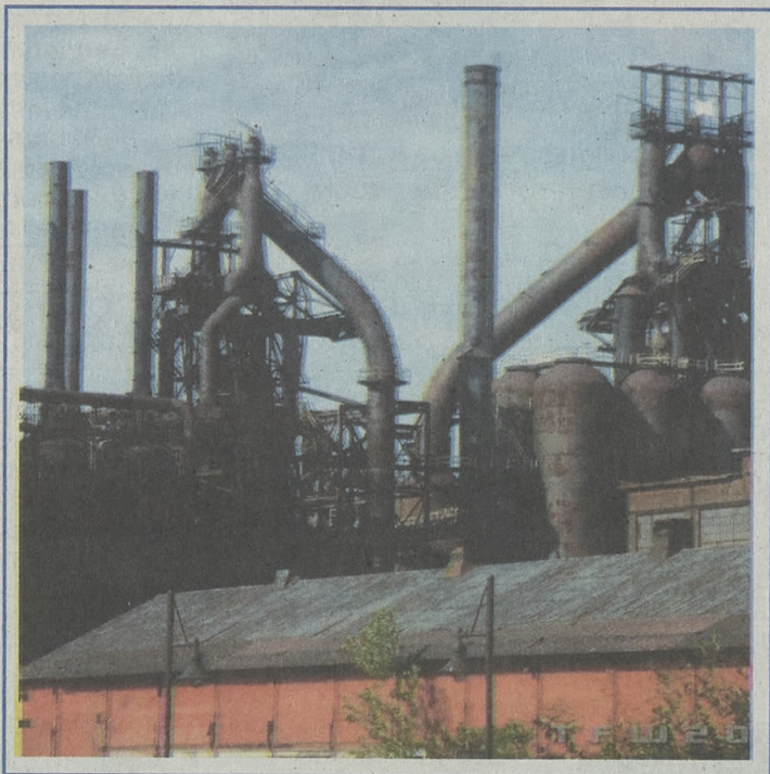
Steel Stacks - Bethlehem
