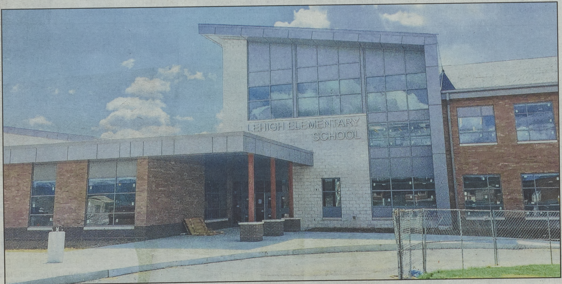
The library is located under a slanted roof on the building's second floor.
