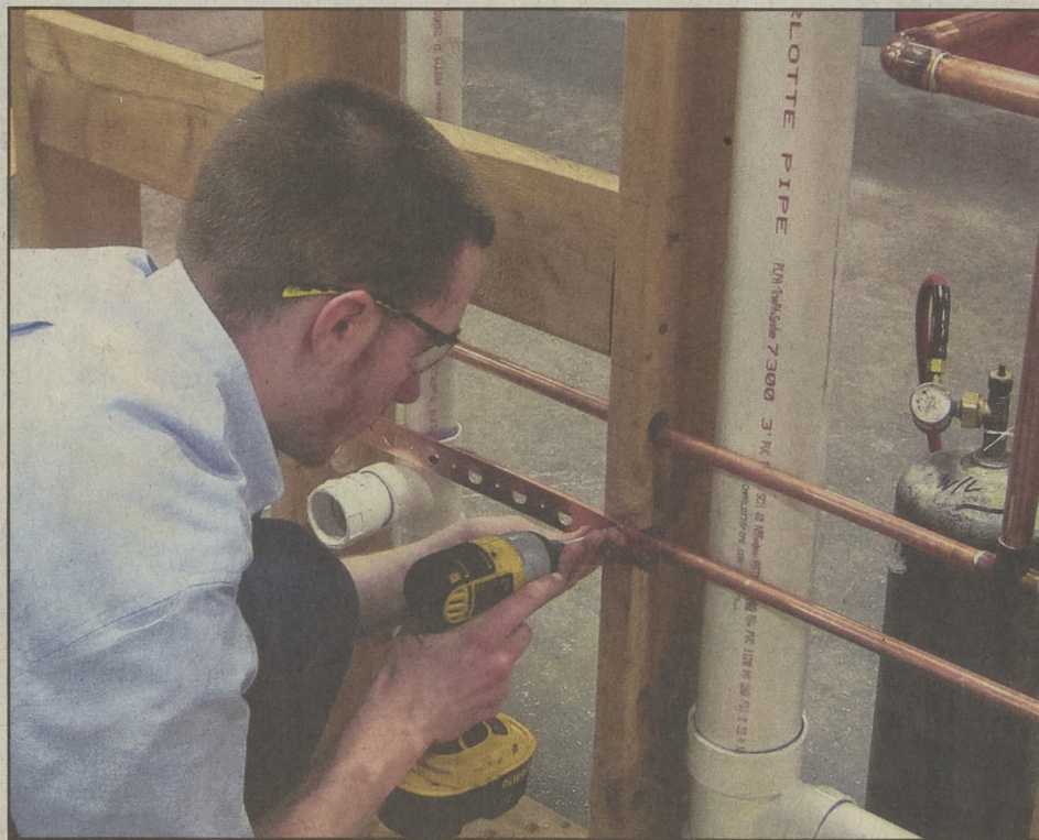
Brandon Kutos, residential plumbing, BAVTS/Freedom (1st Place)
