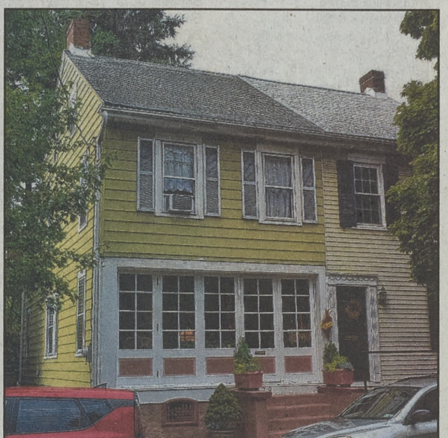
229 E. Church St. was approved for replacement roofing at the Oct. 5 HARB hearing.
