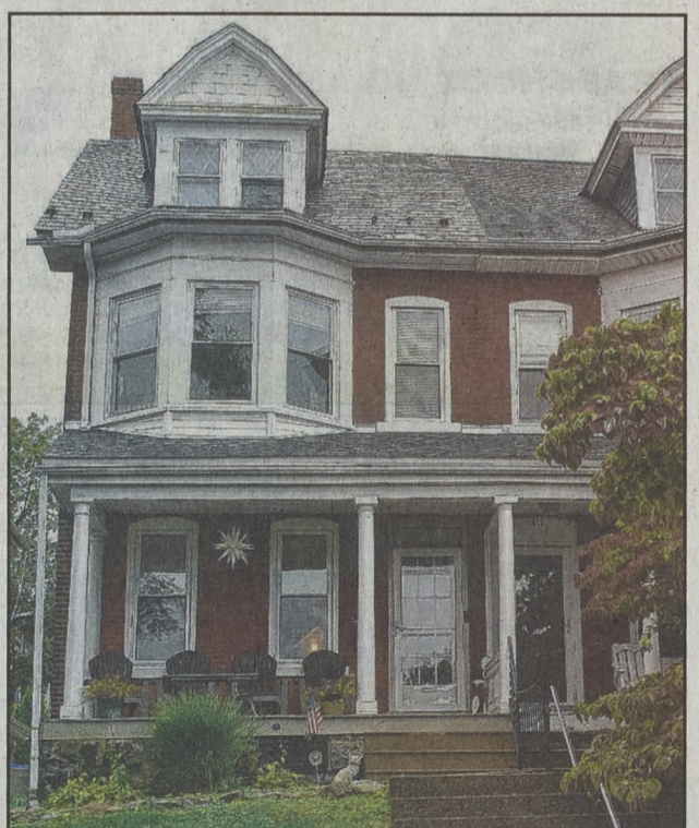
Peter Fox scored a COA to replace the failing slate shingles at 409 First Ave. with GAF Slateline Antique Slate shingles.
