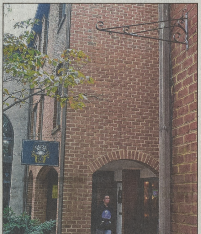
A blade sign for this existing bracket at 77 W. Broad St. #16c was approved at the Oct. 5 HARB meeting for Among Friends, a hair salon. The business faces the Sun Inn Courtyard.
