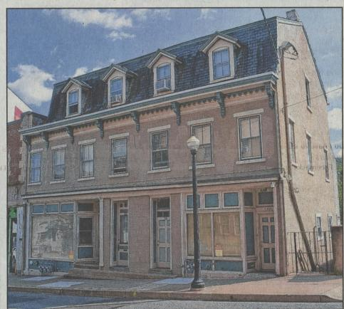
Mark Plosa, owner of 328 - 330 W. Fourth St, was approved to replace worn slate with GAF Slateline shingles, repairing damaged soffit, fascia and trim, as well as repainting the building
