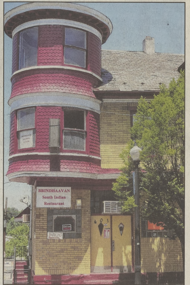
Brindhaavan South Indian restaurant owner Kalavathi Shunmugam suggested extending the existing glass on the door, replacing the window with clear glass and enlarging the window and sign on her restaurant, located at 401 East Fourth St.
