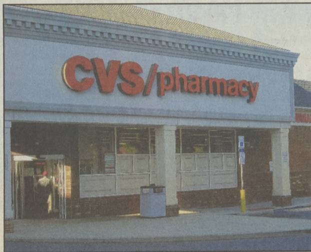
CVS PHARMACY at 305 West Fourth St. got the go-ahead to add historical photographs to existing outside decorative panels.
