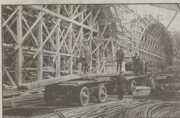
Construction of the Hill to Hill Bridge (1921-1923.)
