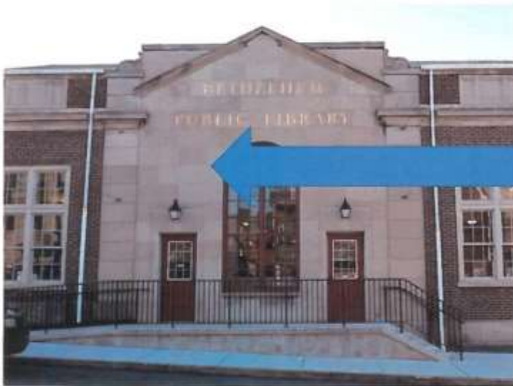
South Bethlehem Library 400 Webster Street
