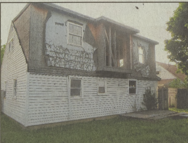
1240 Pennsylvania Avenue, rear view
