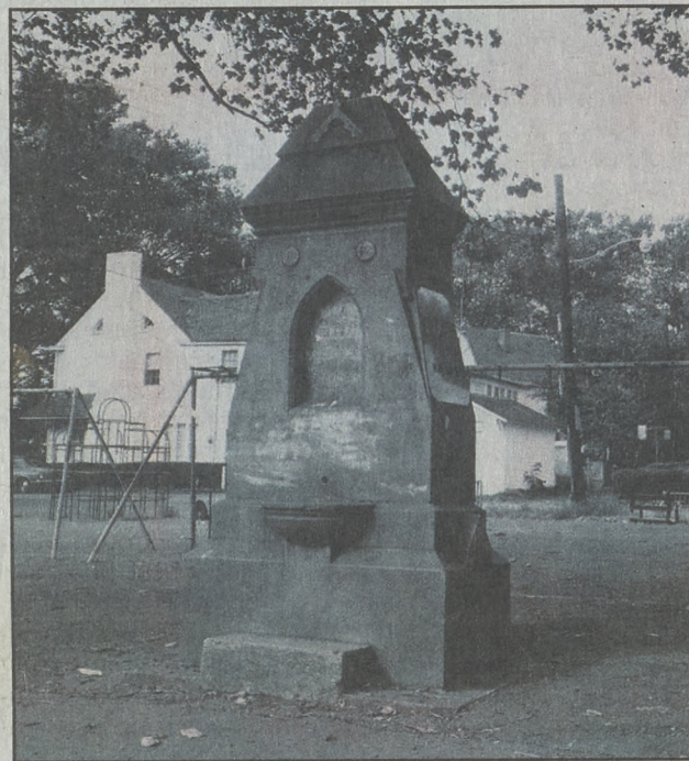
The Eliza Richardson Fountain sits in disrepair at Elmwood Park.
