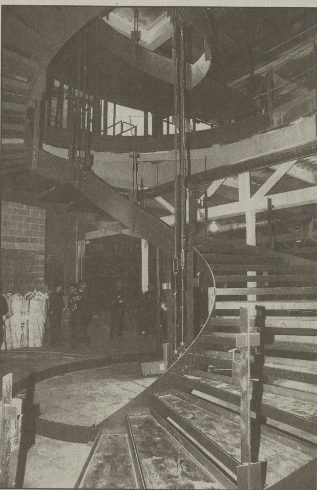
A spiral staircase will take visitors to the arts center between the second and fourth floors.
