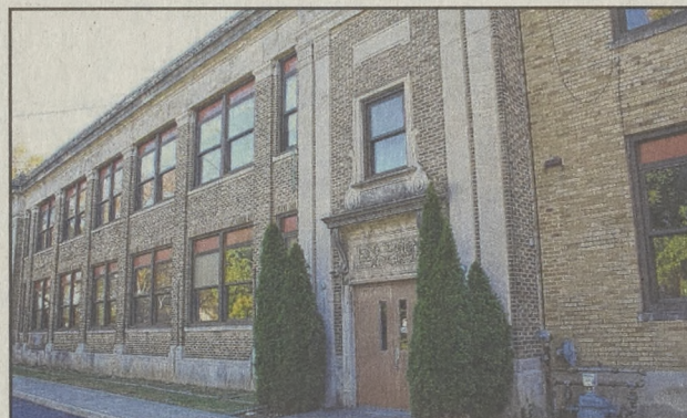
Developer Abe Atiyeh plans to turn the vacant Rosemont ES into a 75-bed assisted living facility.
