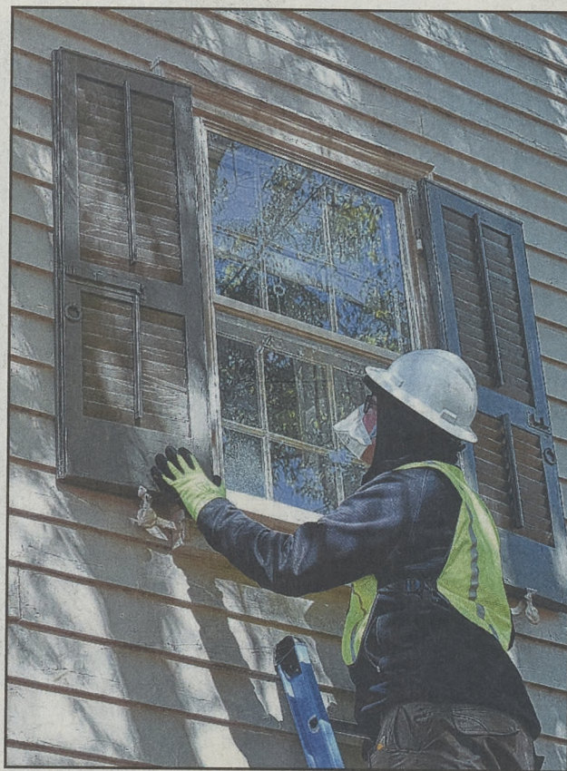
Spencer Jacobsen makes sure the shutter dog is holding the newly-hung shutter in place. "We all have a deep appreciation for history," says Jacobsen of himself and those he works with.
