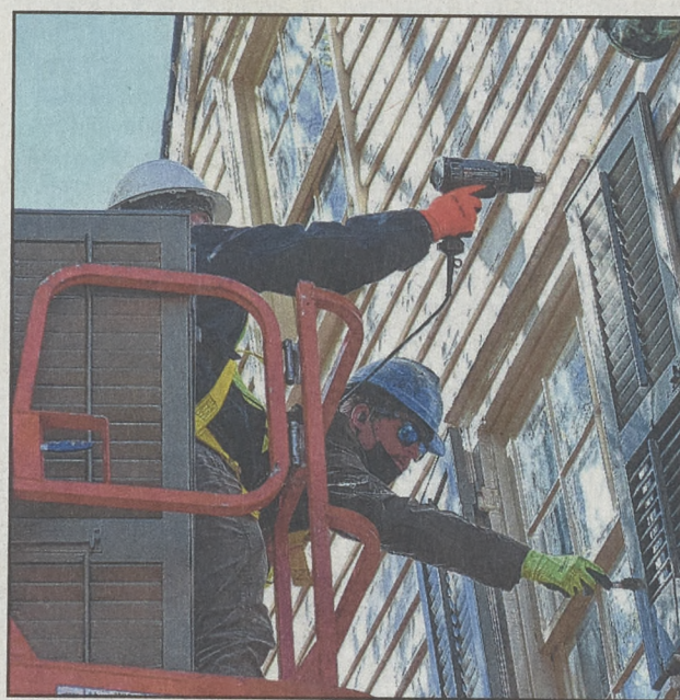
Adam Cygan, touches up paint that had been scratched during transport as his coworker Trevor Ryan dries the wet paint.
