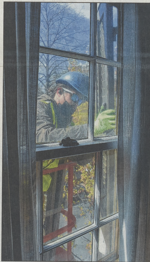
Adam Cygan carefully hangs a shutter on a second floor window.
