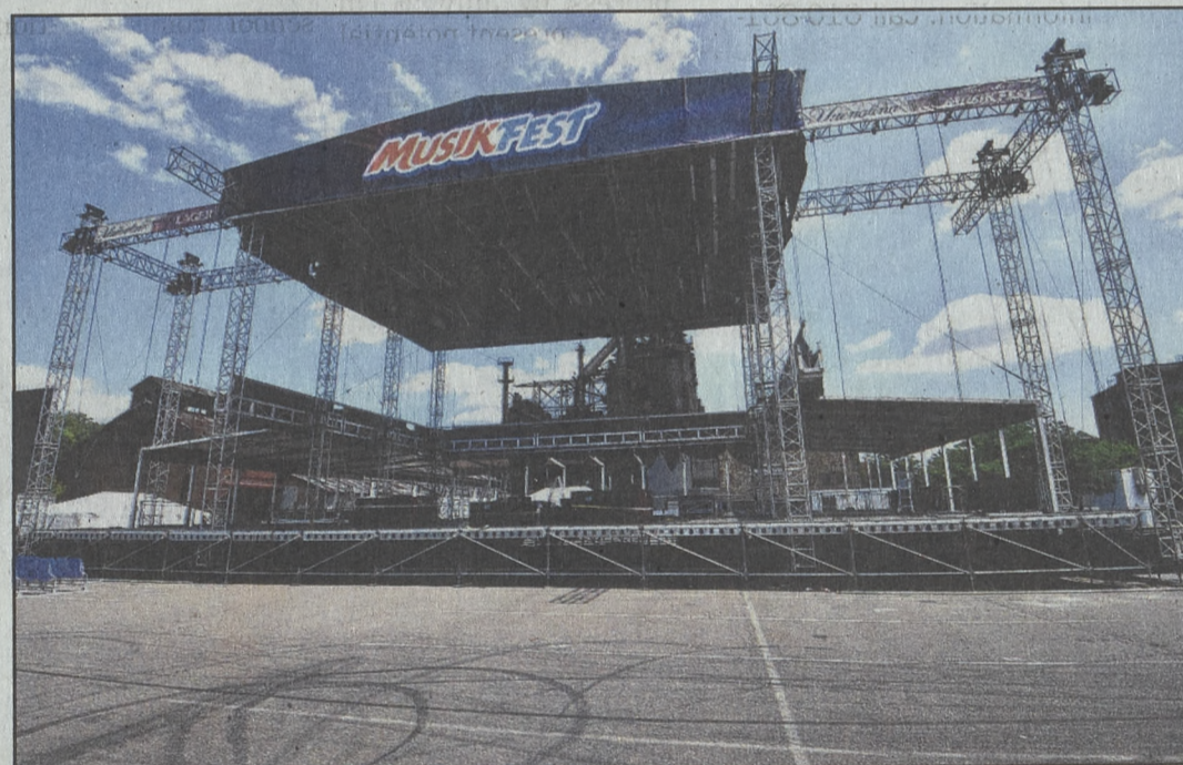
By July 28, the stage roof has been lifted into place.
