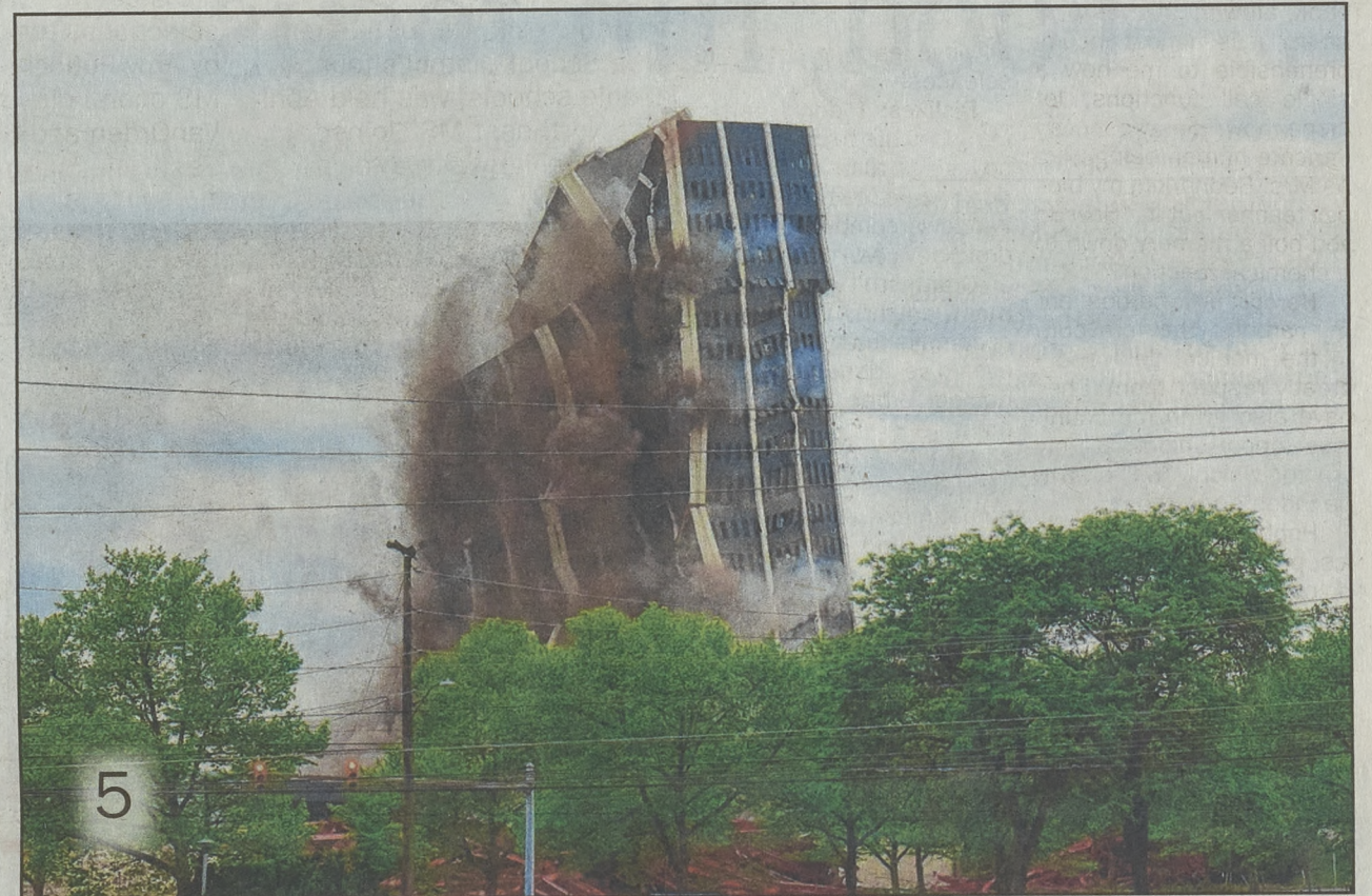
5 The entire Martin Tower collapses into itself.
