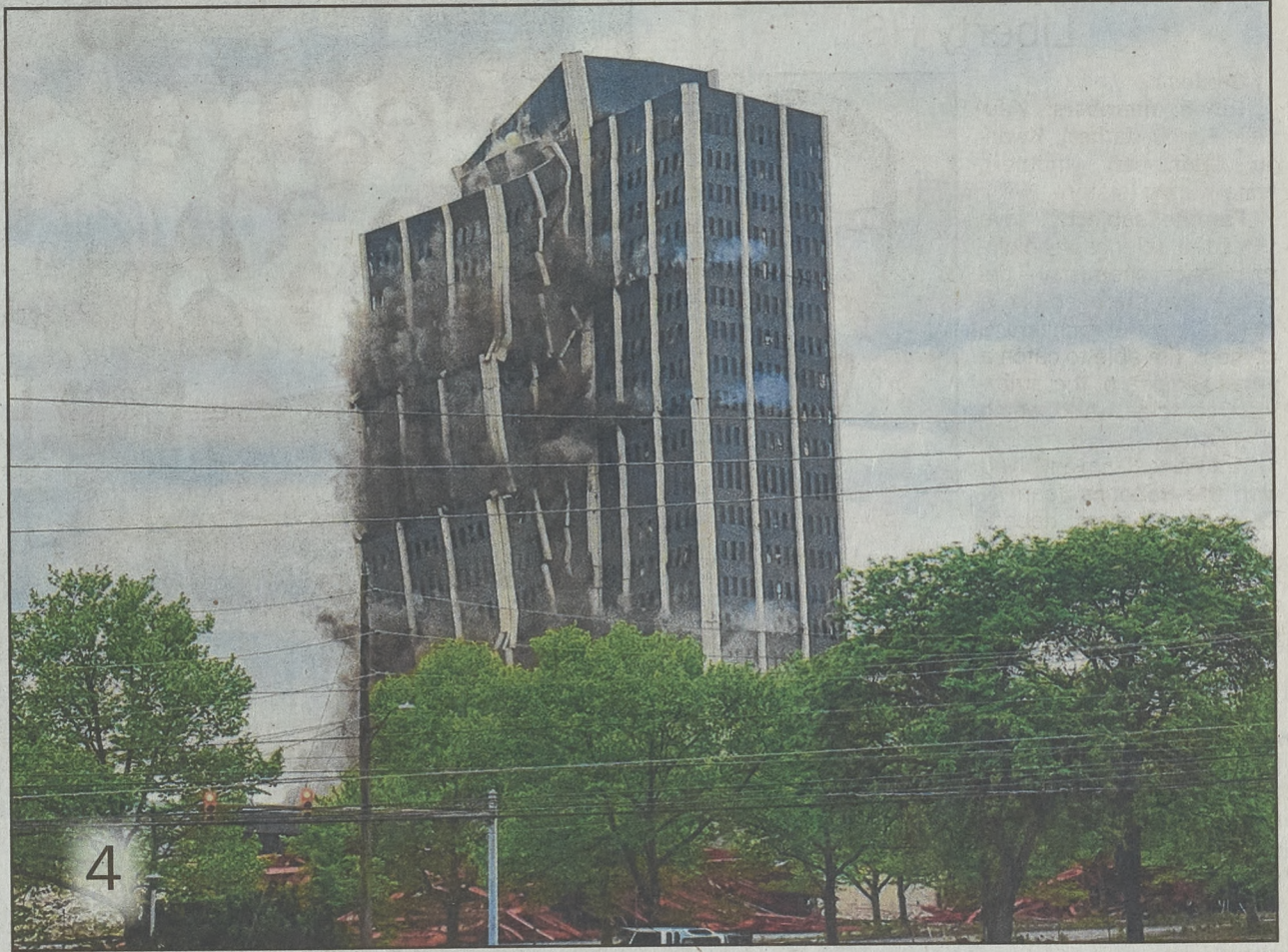
4 As the eastern side slides down, the penthouse begins to collapse.
